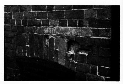
Fig. 8 HYTHE. Brick-tiles side-hung to form arch.
